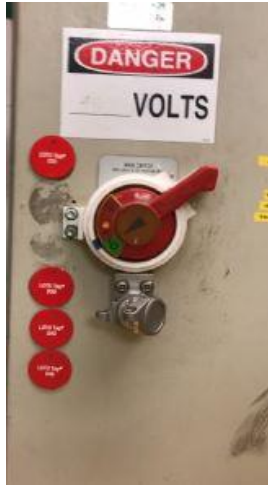
KIRK Applied Engineering Services custom collar solution, installed on customer's equipment, with Type F interlock for power isolation.
