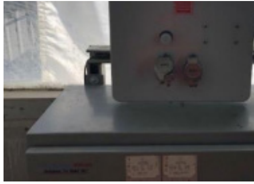
KIRK Type TDKRU time delay unit to ensure residual energy is completely dissipated.
